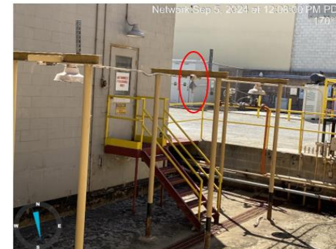
Methane sensor 2 behind the compressor room
