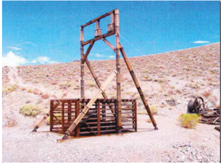
Cupola prevents people and animals from falling into an abandoned mine shaft. Photo courtesy of the California Department of Conservation.
