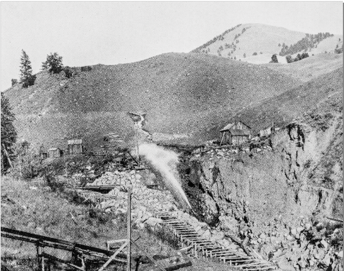
Hydraulic mining caused erosion and increased sediment loads in rivers and streams.
