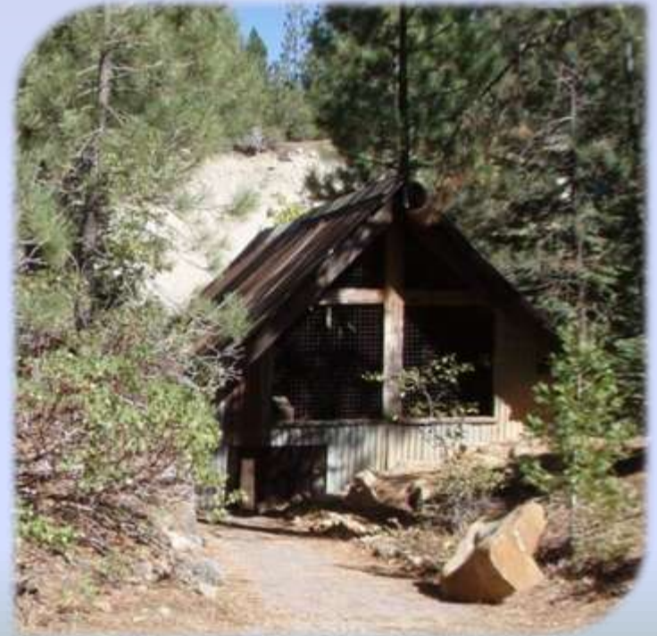
Powerhouse at Picnic Area
