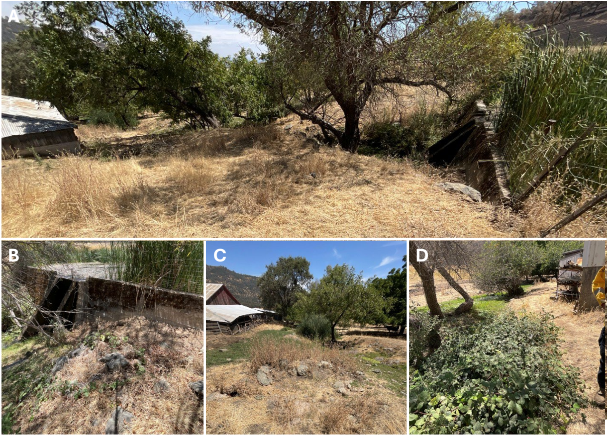
Figure 7. Photographs of VAR #2. A) View looking downstream of B) concrete weir structure. C) View looking downstream showing barn that may be impacted by flooding. D) View looking upstream below most downstream building, which may be impacted by flooding.
