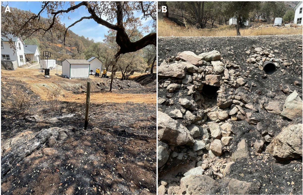
Figure 6. Photographs of VAR #1. A) View looking downstream at channel, house, and outbuildings. Dirt road crossing is a potential location where streamflow could overtop the stream left channel bank and flood the house and outbuildings. B) Looking upstream at outlets of 16" (left) and 12" (right) culverts downstream of the house. These culverts may become plugged, and the driveway could become flooded and damaged.
