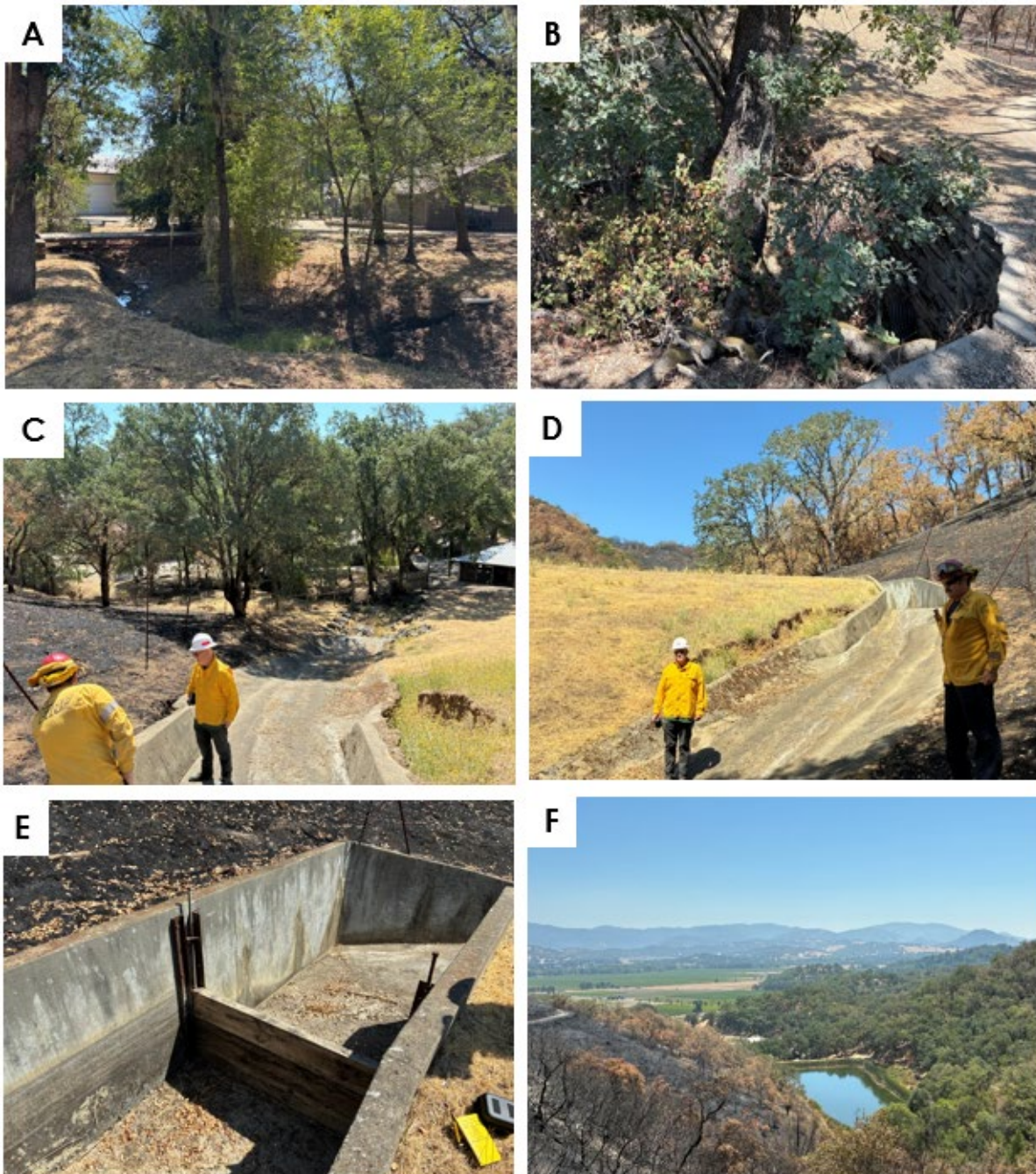
Figure 6. Photographs of VAR #1. A) View looking downstream at channel and outbuildings. B) 48" CMP at road crossing downstream of Photo A. C) Spillway transitioning to natural channel, with sharp left-hand turn in channel next to pumping station (right). Note scour of dam material adjacent to spillway. D) Dam face and spillway. Note scour of dam material. E) Wooden floodgate structure consisting of removable planks at crest of spillway. Notebook at right of image is located on dam crest. F) View of pond, dam, and structures from upper watershed.
