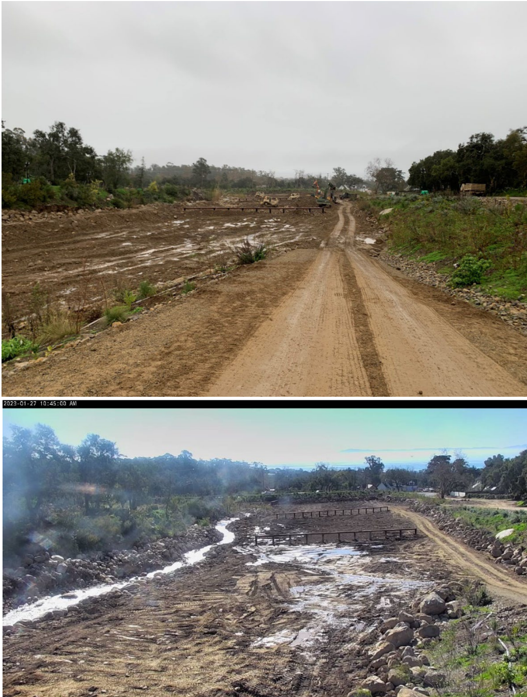
Figure 6. Photo of CNG actively excavating material from basin on January 14, 2023 (Top) and basin completely empty of debris and returned to near-previous conditions on January 23, 2023 (Bottom)
