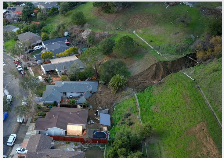
A home impacted by a rainfall-triggered slope failure. The landslide occurred naturally, and its impacts might be reduced through planning or engineering. Photo credit: Hayward Police Department.
