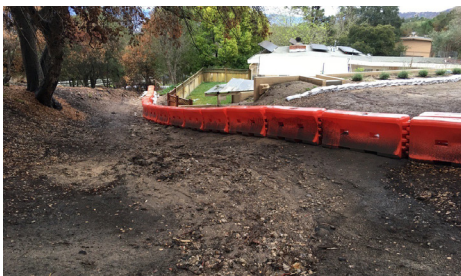
Temporary barriers deflect flow and debris.
