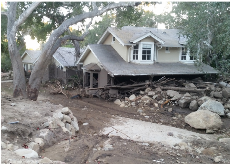
Damage from a major debris flow in Montecito, CA, after the 2017 Thomas Fire.
