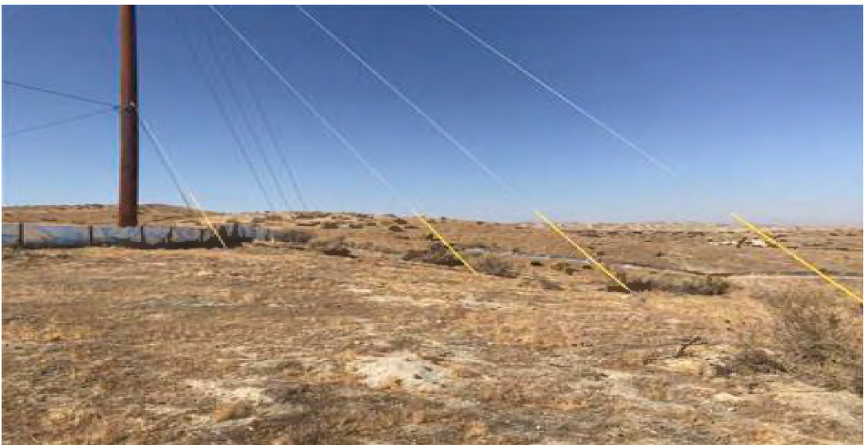
Photo 12: View of well pad location 616-12D and surrounding area. GPS Coordinates: 35.155121, -119.357370, facing east. Taken by Karissa Denney on October 4, 2022.
