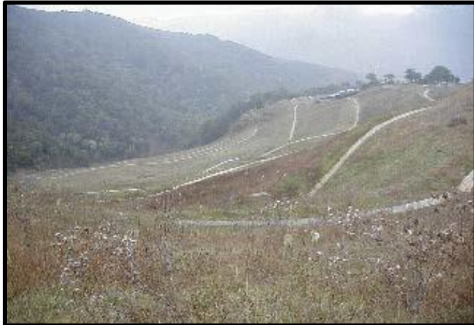
Gambonini Mine final grade with drainage ditches and native vegetation. Photo: DOC (2005)
