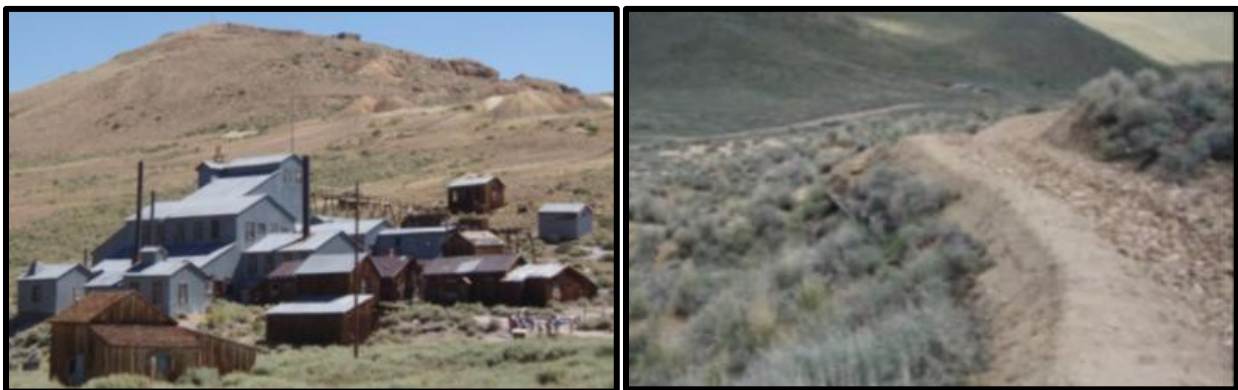
Left: Standard Mill at Bodie State Historic Park. Right: A lined diversion ditch prevents runoff from reaching and eroding mine tailings. Photo: DOC (2009)
